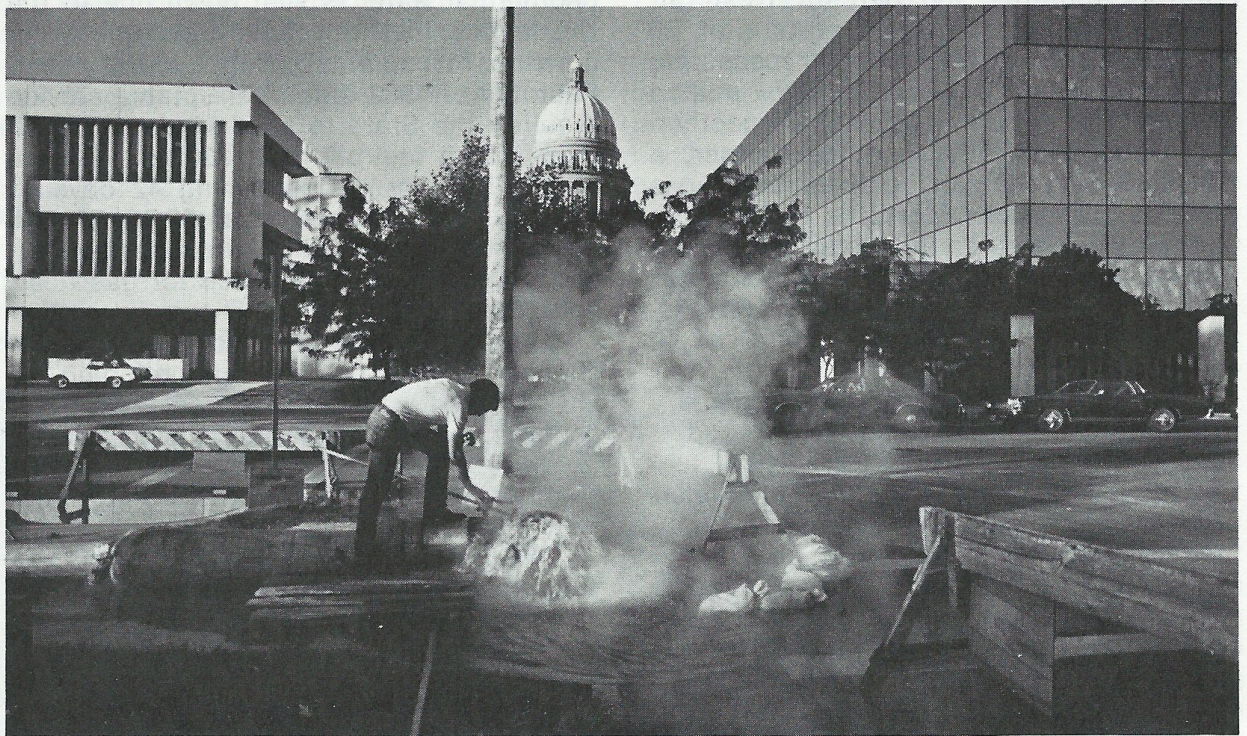
The State of Idaho production well with the Capitol Building framed by two State office buildings. Tests in August, 1981, proved this resource to run 810 gallons per minute artesian flow at 160 degrees.
